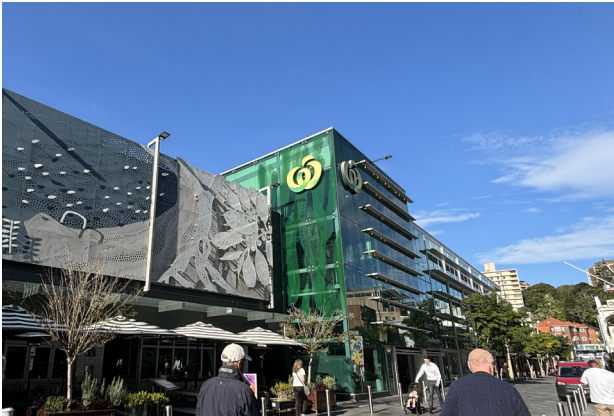
Woolworths frontage / materiality on Kiaora Lane
